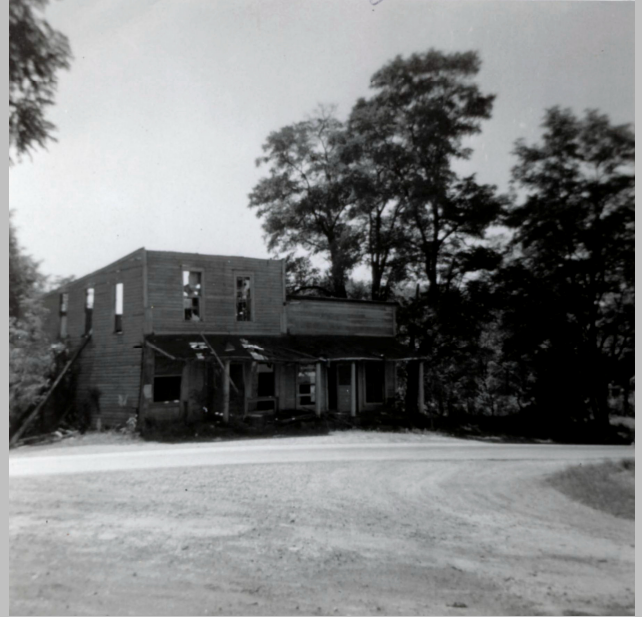
This shows the front of the old store building as it was being demolished, about 1956. It can be seen that there were actually two buildings joined together.
