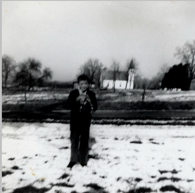
Taken in our front yard (perhaps 1953 or 1954), this shows the church and school. The latter is nearly hidden behind the evergreen trees on the right. Highway 246 is behind me. Both buildings were visible from our front door, so we knew when something was going on! The spreading tree on the left is near the site where "The Famous Newport Shows" made their winter quarters. It was a traveling carnival-like sideshow, operated by the Newport family of early Vandalia (the parents of "Ivy" Newport Jennings and "Theo" Newport).
